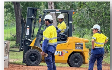
Jeremy using forklift to move cement blocks
